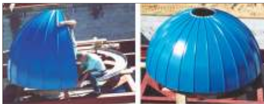
Figure 5. Installation of Curved Dome Panels
