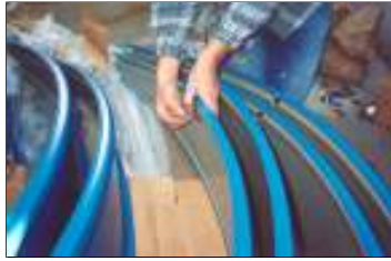
Figure 7. Dome Pane Attachment with Clip and Bolt
