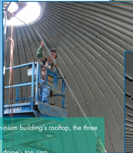
(Middle) A worker installs material over a 4-foot opening at a dome's top ring.
