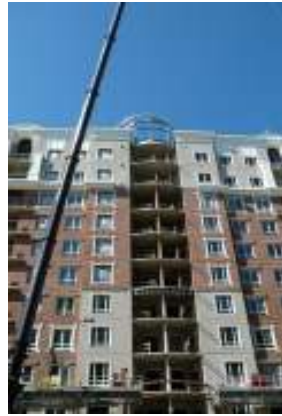
The structure is complete, ready for the dome to be placed.
