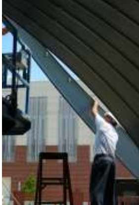
Domes are assembled one panel at a time, with a crew of 3 or 4, depending on dome size.
