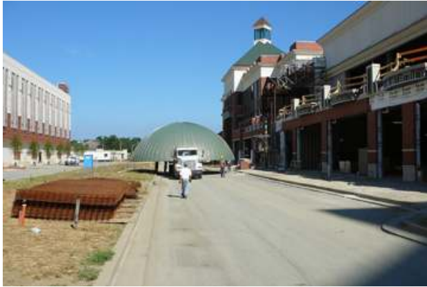
One of three domes en route to the lift site, about 1/4 mile away from the assembly site.
