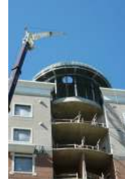
One of the three domes settling into position.
